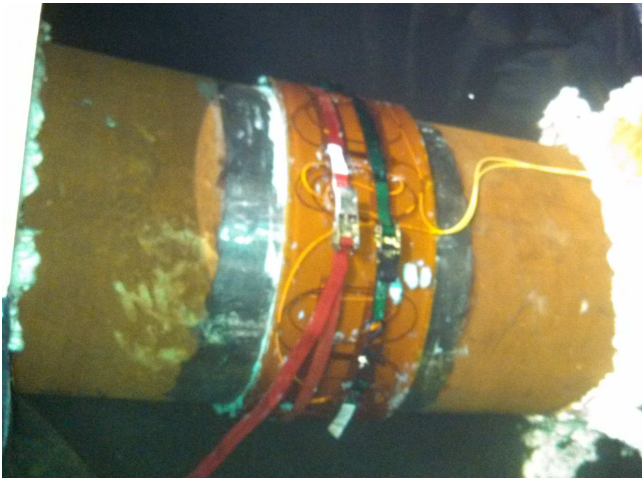
FIGURE 2. INSTALLED CLAMP AND FIBER OPTIC SENSOR STATIONS.
