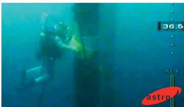
Clamp Installation
