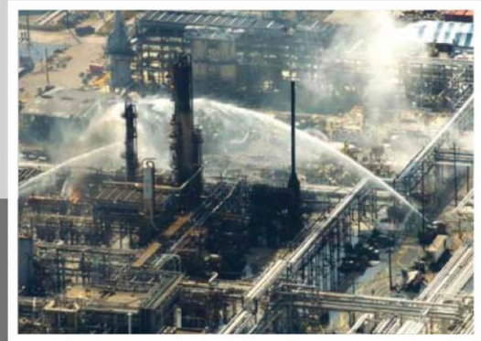
Texas City Refinery 2005
