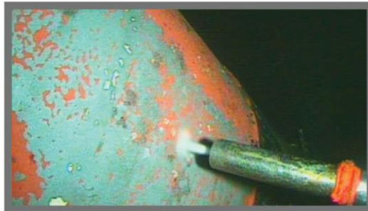
Cleaning with Water Jet
