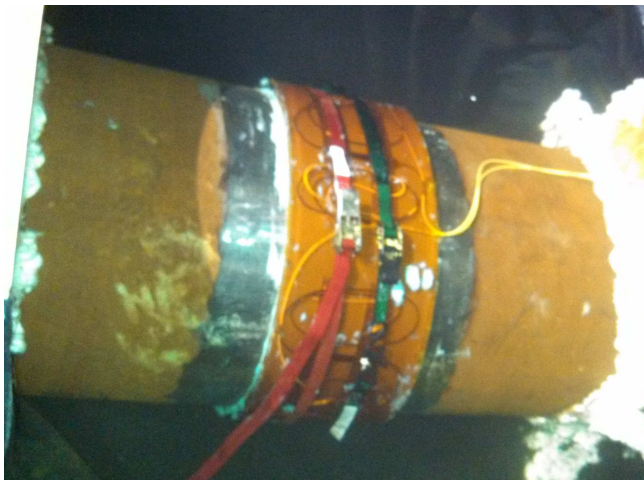
FIGURE 2. INSTALLED CLAMP AND FIBER OPTIC SENSOR STATIONS.
