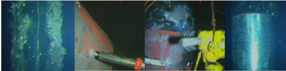
Figure 8. Tendon Preparation for Adhesive Clamp Bonding.
