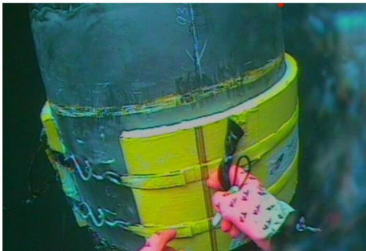
Figure 9. Installation of Adhesive Clamp on a TLP Tendon.
