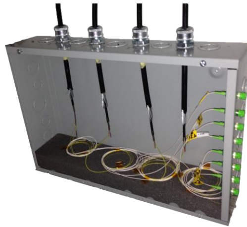
Figure 10. Field Termination Box with 4 Fiber Optic Cables and 8 Interrogation Lines.
